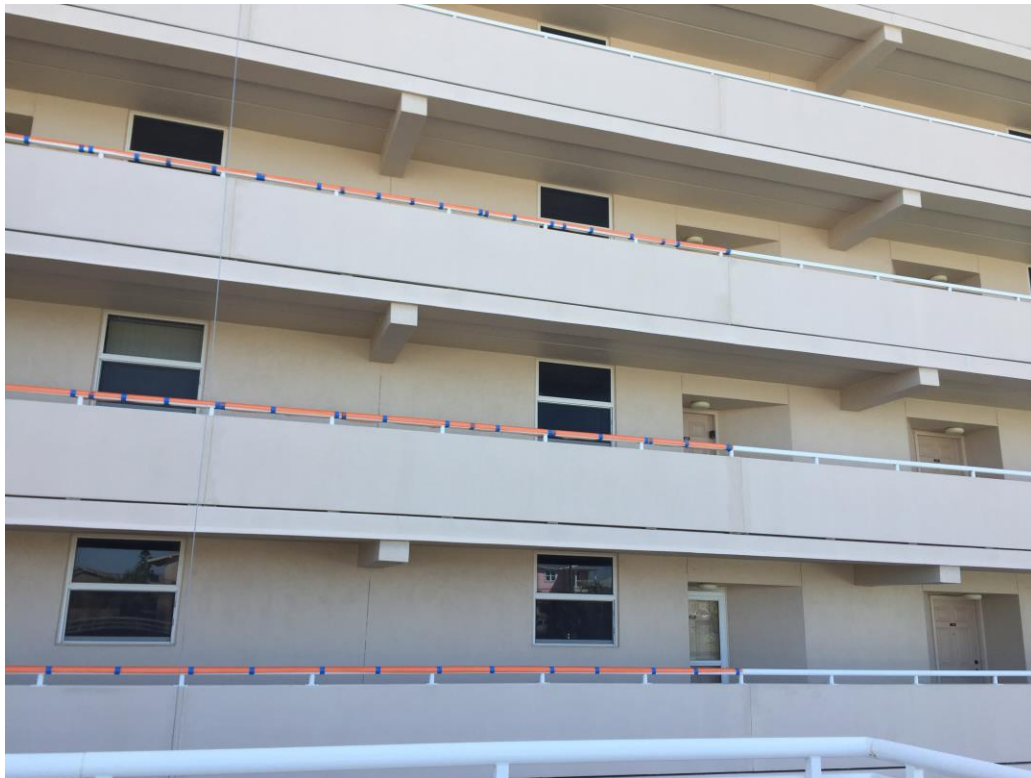
Picture 2: In-progress protection of the walkway guardrails
