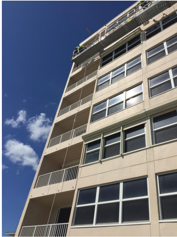
Picture 3: Swing stage mobilized on the 11 stack balconies
