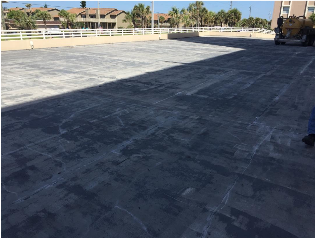
Picture 1: Topside of the parking deck
